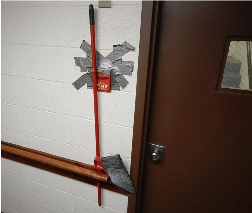
“Example of a patchwork fix actually orchestrated by the fire marshal himself to keep the building operational when a resident pulled the fire alarm and the whole device came out of the wall.”
