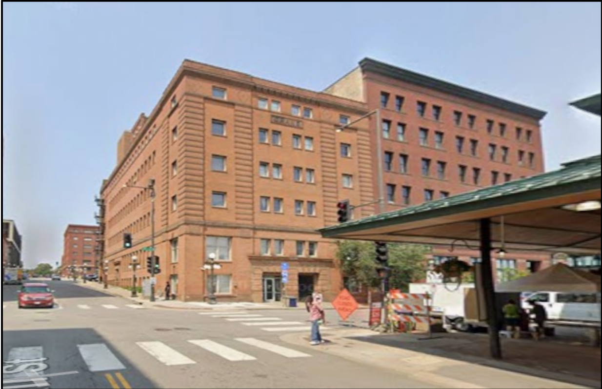
Photo of Crane Ordway Apartments - St. Paul
