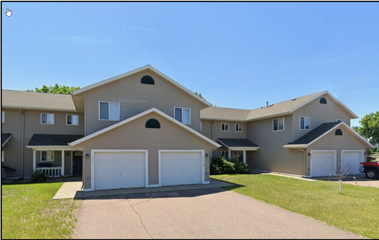
Photo of Rock Creek Townhomes – Luverne
