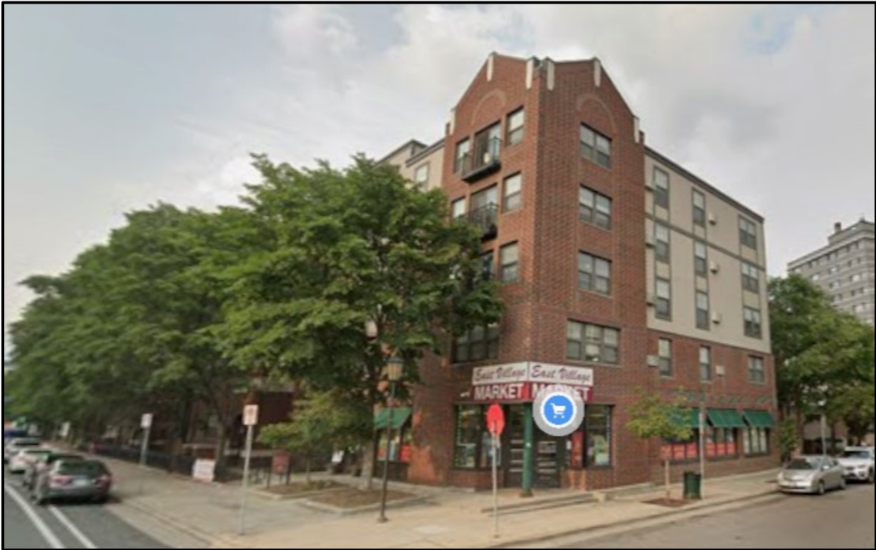
Photo of Endeavors Apartments - Minneapolis
