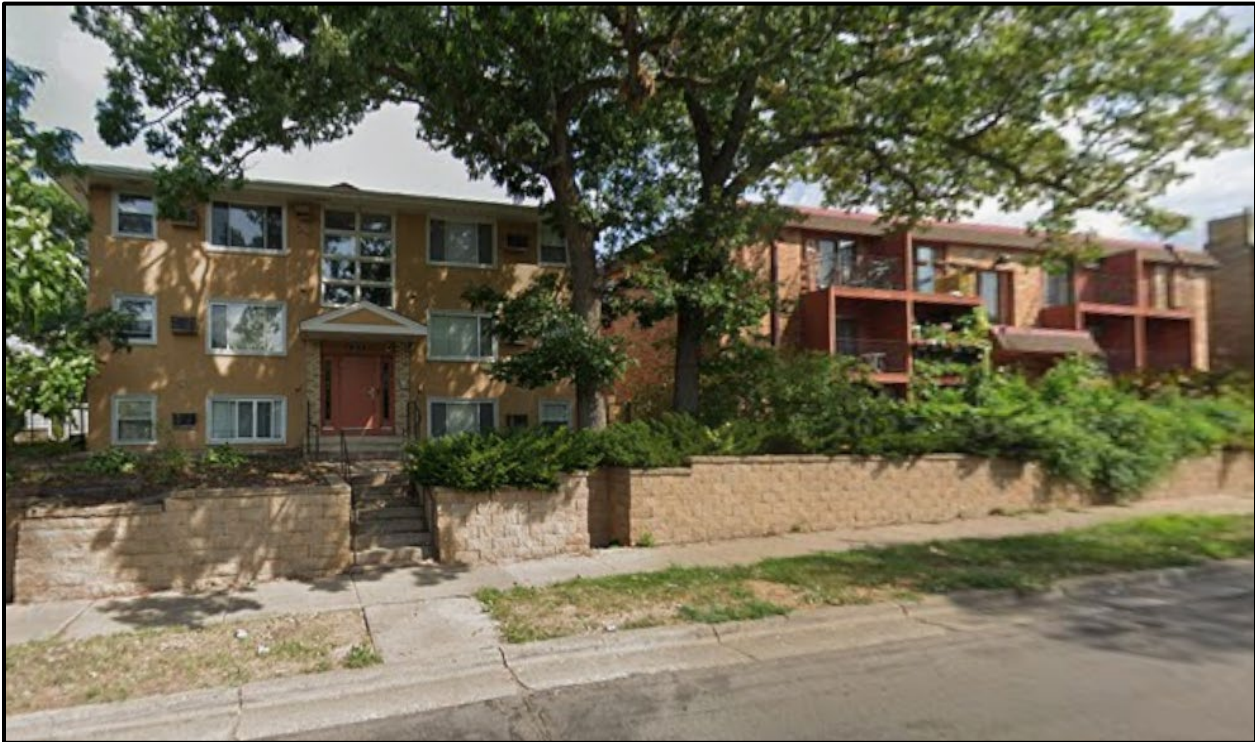
Photo of Dillon Apartments – Minneapolis
